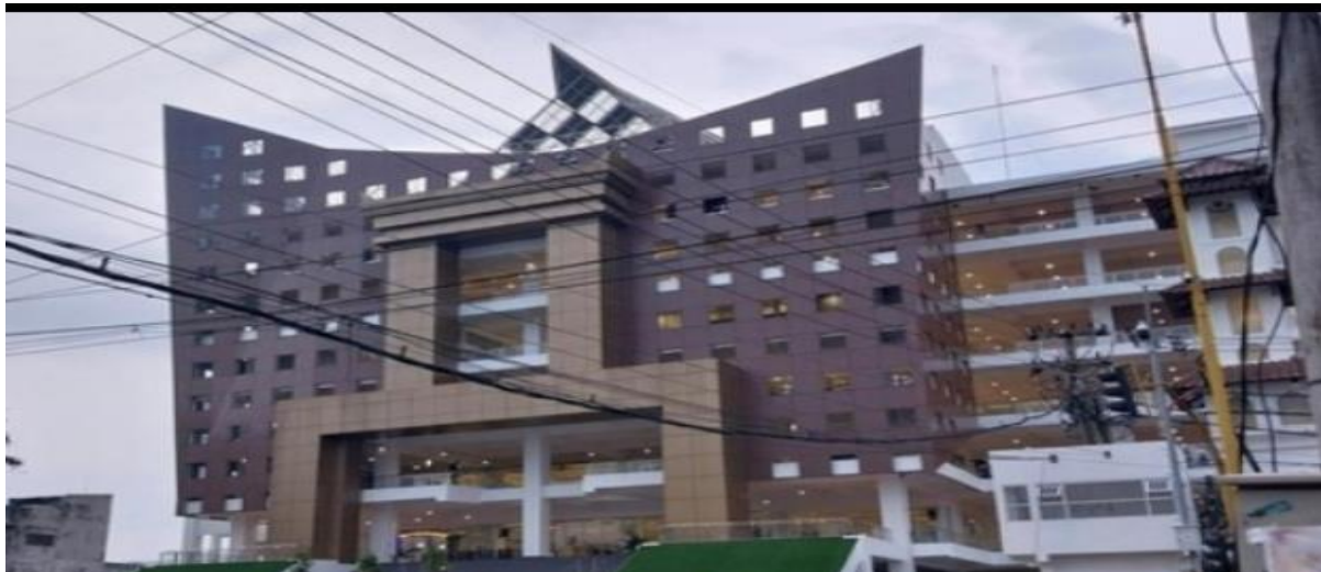
Figure 3. MCC Building (Malang Creative Center) is one form of the contribution of the Malang City Government in managing and maintaining the Creative Economy ecosystem, as well as a forum for EKRAF actors to collaborate and grow together between Creative Industries.
