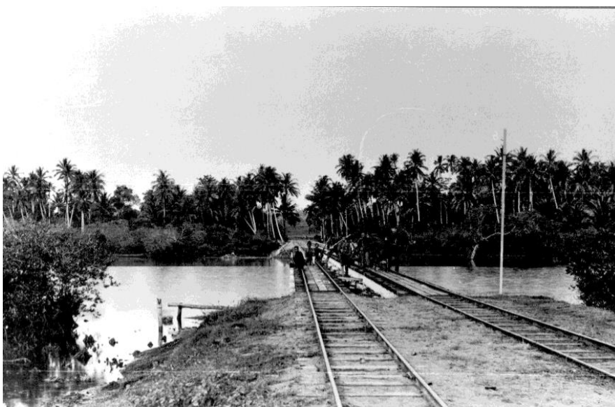
Figure 1. Two railroads over the river in Lhokseumawe built by the Dutch in 1930 (Source: ANRI, KIT Aceh No. 0093/022)
