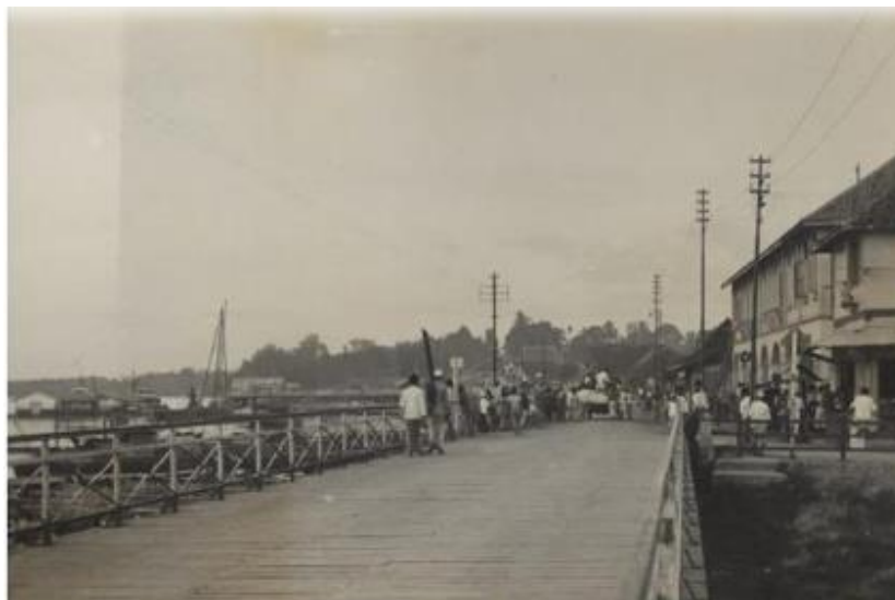
Figure 1. Batu Boom Pier Source: Saputra et al., 2023
