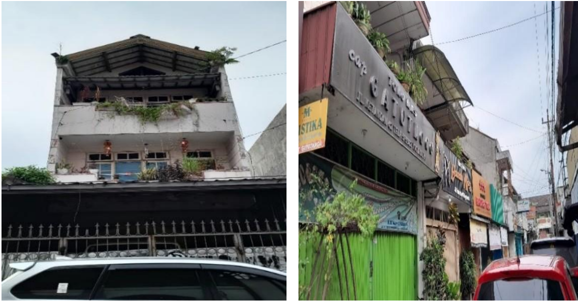
Figure 1: Architectural forms in Ketandan Village Source: Personal Documentation, March 10, 2024
