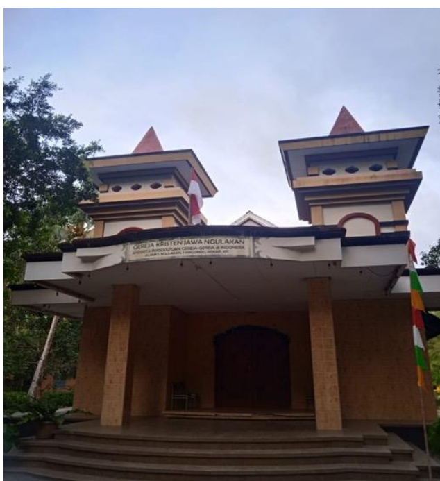
Figure 1: The GKJ Ngulakan Church Building (Post-Renovation)
