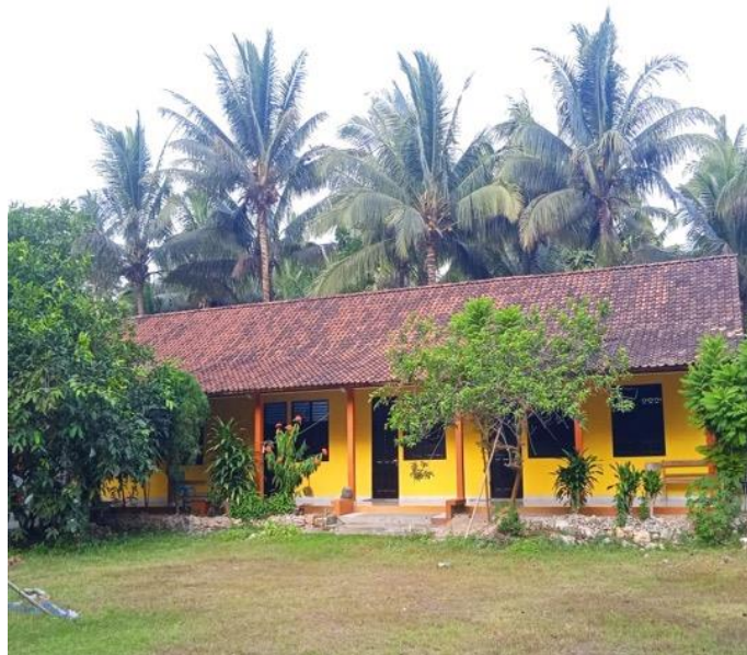
Figure 2: The Bopkri School Building (Post-Renovation, April 14, 2024)
