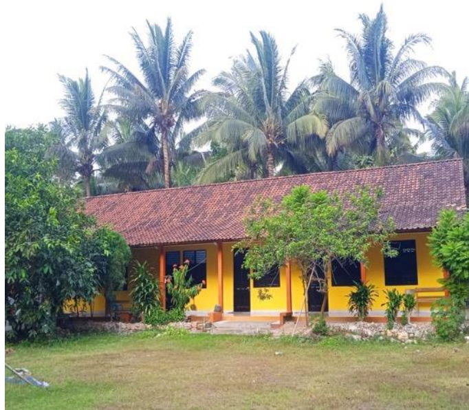
Figure 2: The Bopkri School Building (Post-Renovation, April 14, 2024)
