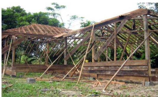
Figure 2. Frame Structure of a Transmigrant Farmer's House Source: Processed from the Archives of DPW SPI Jambi
