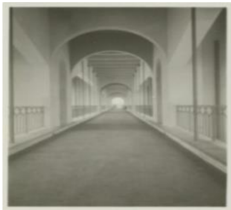
Figure 1. Walahar Dam, Karawang, interior view
