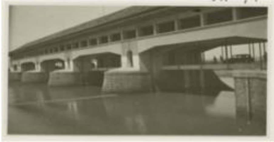
Figure 2. Walahar Dam, Karawang, 1931
